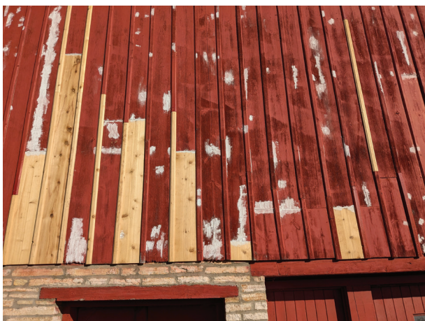
Board and batten siding repair and replacement
