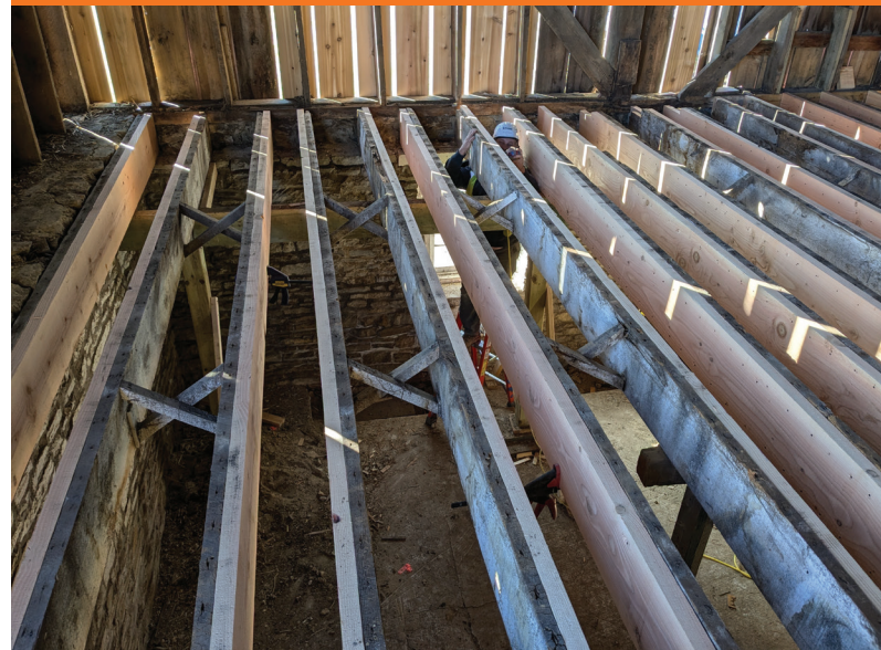
ABOVE: Sistered joists at the southeast bay of the barn BELOW: Structural engineer’s diagram, Benjamin A. Wolf, PE (IA, MN, WI), Short Elliott Hendrickson, Inc.
